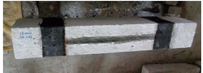
Fig -5: RC beam with CFRP U –wrap provided as end anchorage for NSM system
