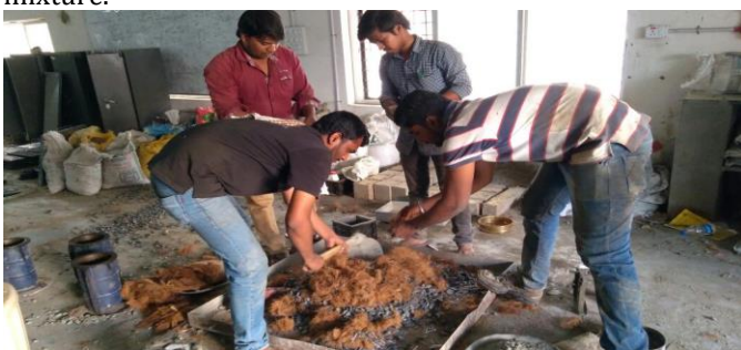
Figure 4.4: mixing of concrete
