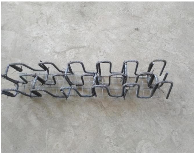
Figure.6. Reinforcement used in Ferrocement Concrete Beam
