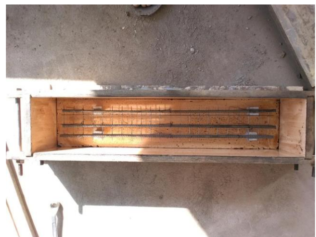
Figure.4. Reinforcement with Mould
