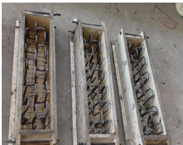
Figure.6. Setup for Ferrocement Concrete Beams
