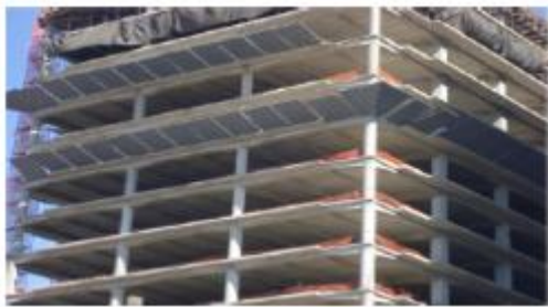
Fig -2: Ribbed slab system
