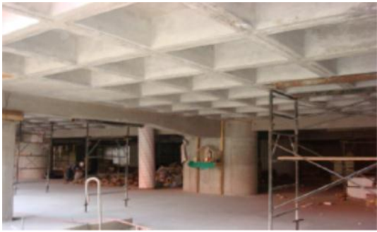
Fig -1: Waffle slab system
