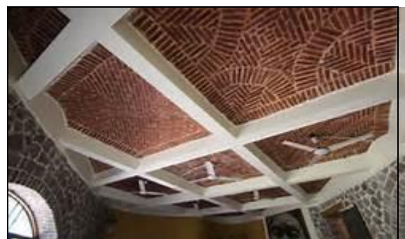
Fig-1: Typical view of Funicular Shell roof.
