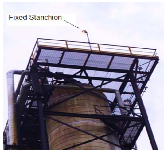
Fig-2: Light fixture maintenance at heights
