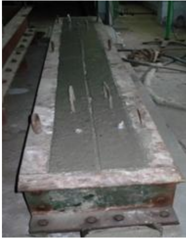
Fig. 2 Pretensioning of GPC Sleepers
