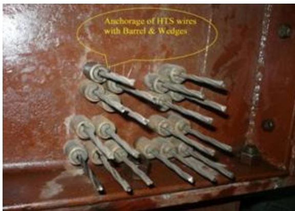
Fig.3. Anchored in HTS Tendons with Barrel and Wedges
