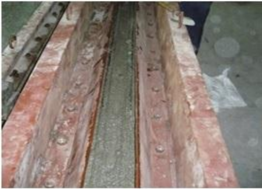
Fig.4. Casting of Railway Sleepers
