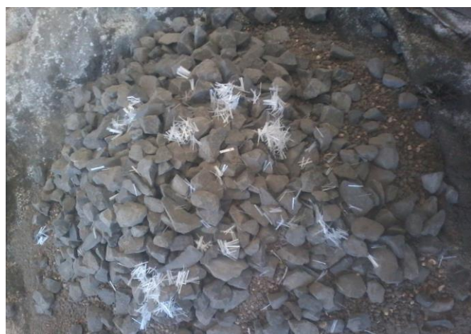
Photograph No: 6 (Casting of concrete with polypropylene fibre)
