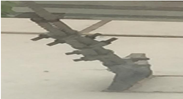
Fig -5: Fixing tendon at corners of frame
