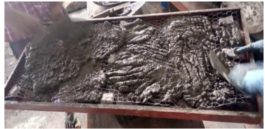
Fig - 4: Casting of rectangular panel.
