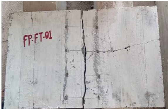
Fig. – 6: Crack pattern of RP-01
