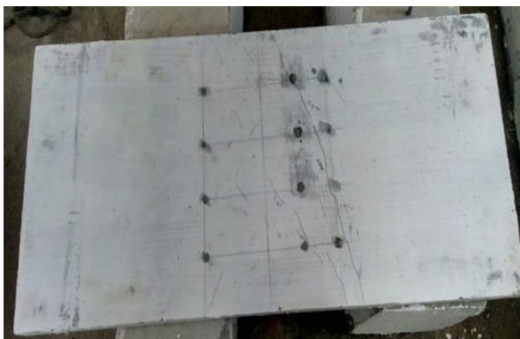
Fig – 8: Crack pattern of RP-03
