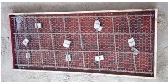
Fig - 3: Fabrication of mould
