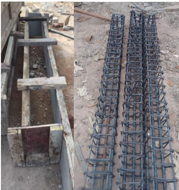
Fig-5 Form work and reinforcement cage for three beams
