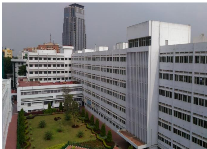
Fig -1: Building taken up for survey
