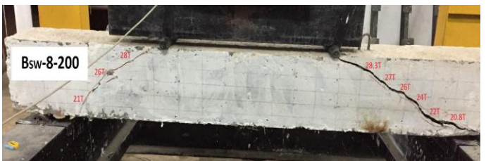
Fig -11: Crack pattern of BSW-8-200
