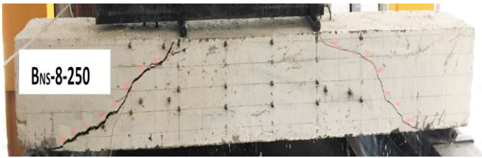
Fig -7: Crack pattern of BNS-8-250
