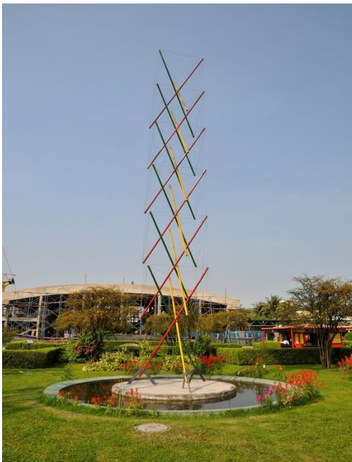
Fig.1 12m high tensegrity structure exhibit at the Science City, Kolkata.
