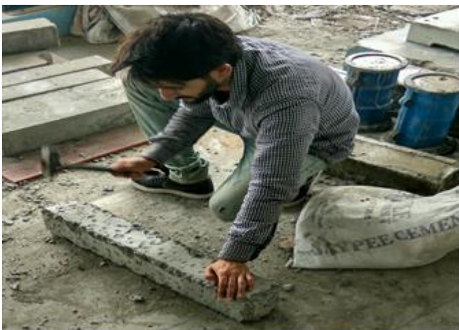
Fig - 2 Preparation of surface of columns
