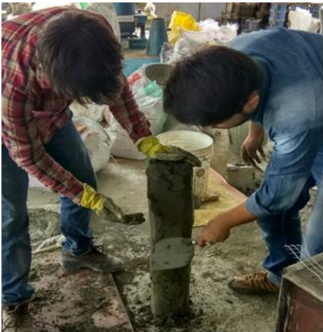
Figure 4 Application of ferrocement matrix
