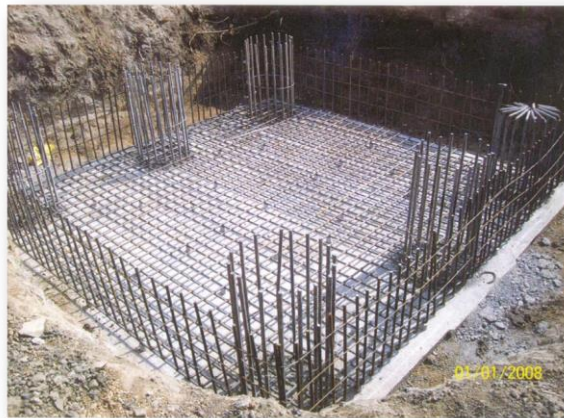
Fig 4.1: Foundation of pier
