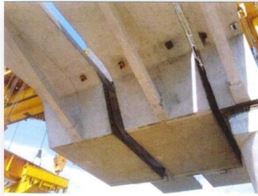
Fig - 4.6: Placing of segment in order
