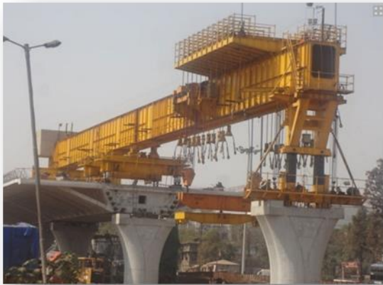
Fig - 4.5: Segment being lifted and placed
