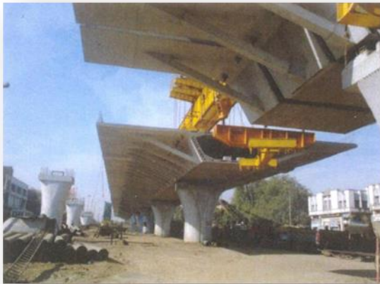
Fig - 4.5: Segment being lifted and placed
