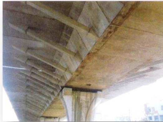
Fig - 4.6: Placing of segment in order
