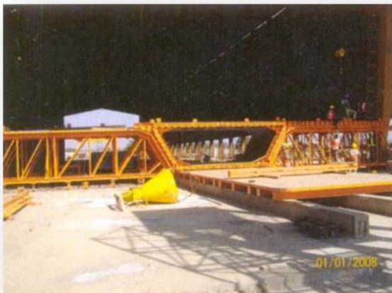
Fig - 4.4: Formwork of the Segment at the casting yard Fig - 4.5: Segment at the site yard
