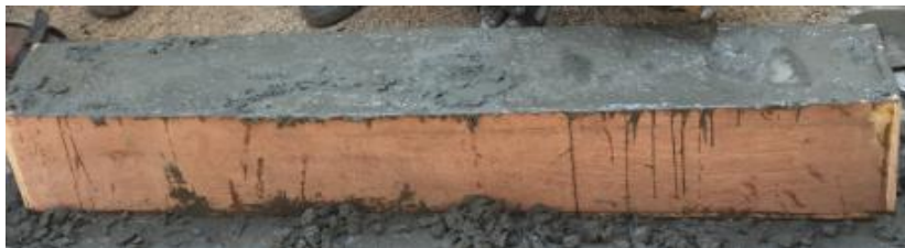
Figure 2: Casting of Control Beam
