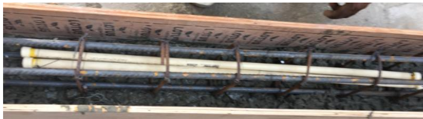
Figure 3: Casting of Replaced Beam
