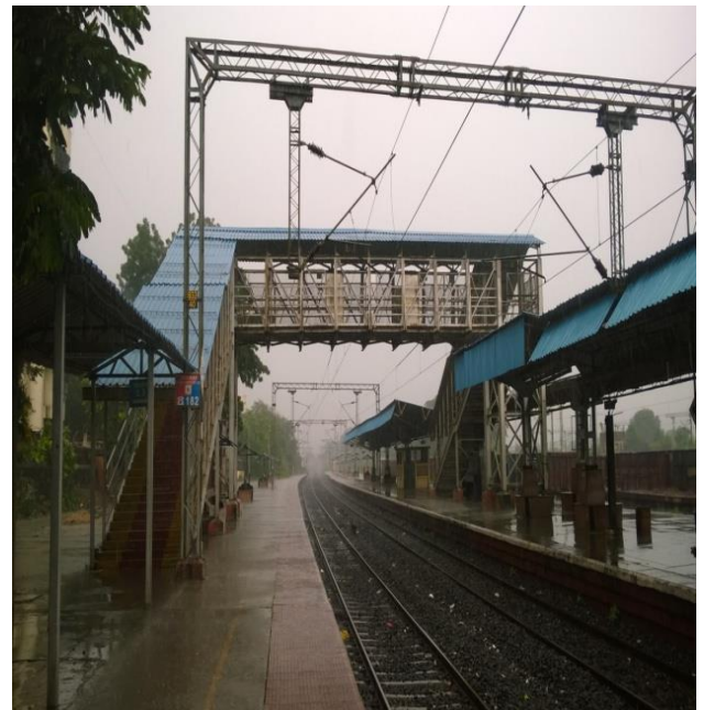
Fig.:- Foot Over Bridge
