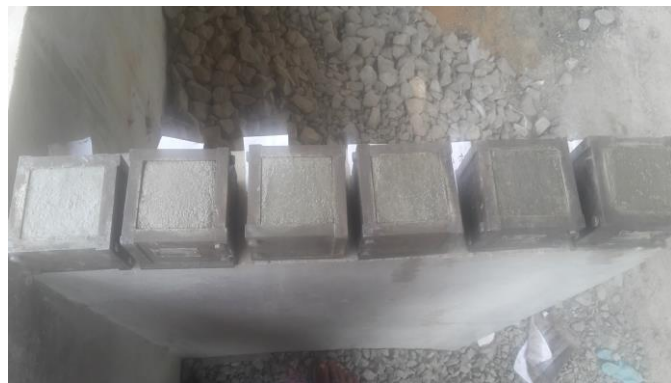
Fig -3: Casting of cubes
