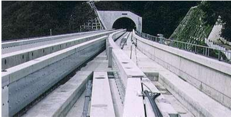
Fig 15 Turnout Facilities of the Maglev Test Line
