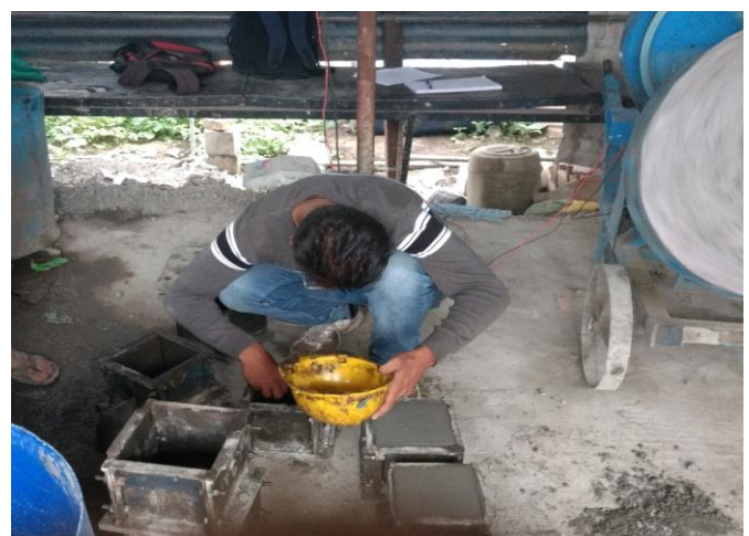
Fig No.:-2.1 Showing final finishing of casted cubes
