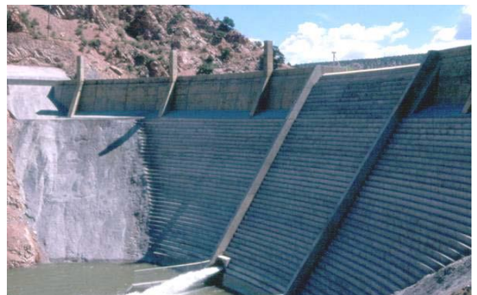
Figure. 1 RCC SANTA CRUZ DAM
