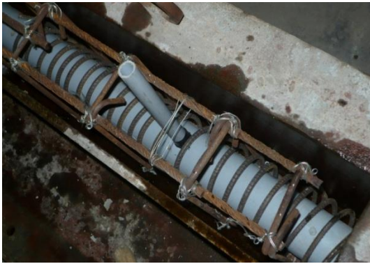
Fig.17. Casting of Post-tensioned Beam
