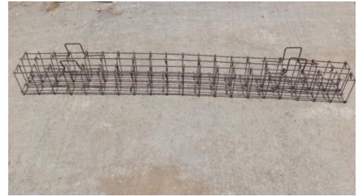
Fig.1. Arrangement of Reinforcement grill
