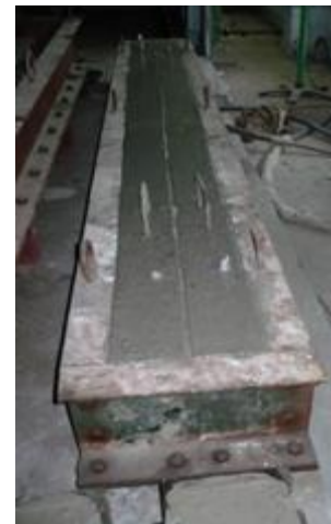
Fig.2. Casting of Concrete Beam
