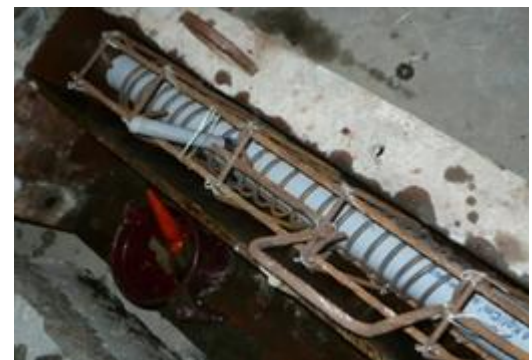
Fig.16. Mould with spiral end anchorage
