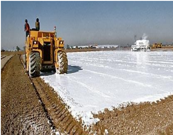
Fig-1: Lime Stabilization
