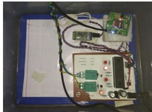
Fig 12: View Of Receiver
