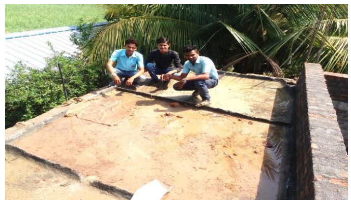
Fig.1 ponding and immersion
