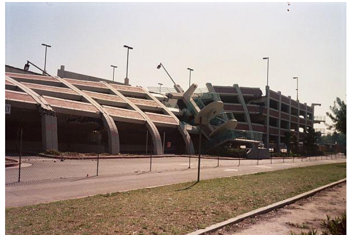
Fig.1: Structural collapse due to effect of P-delta
