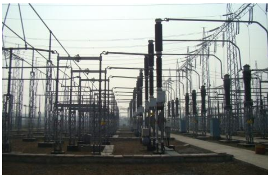
Fig.1:- Constructing the New Substation.
