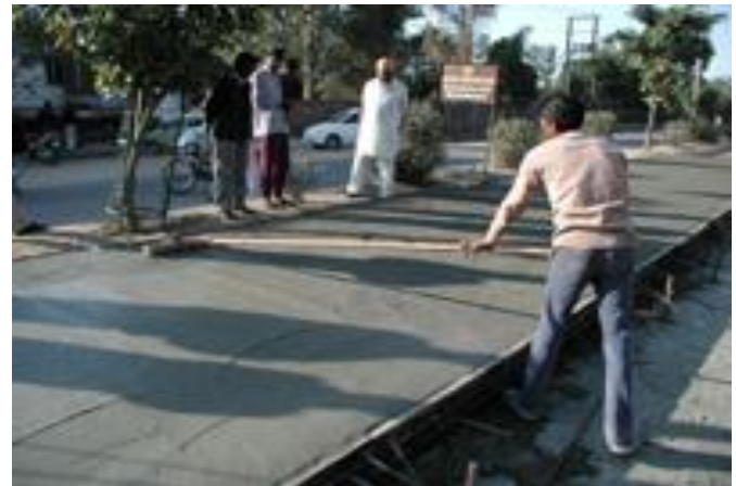
Fig 3 TYPICAL CONSTRUCTION OF ROAD USING HVFA CONCRETE
