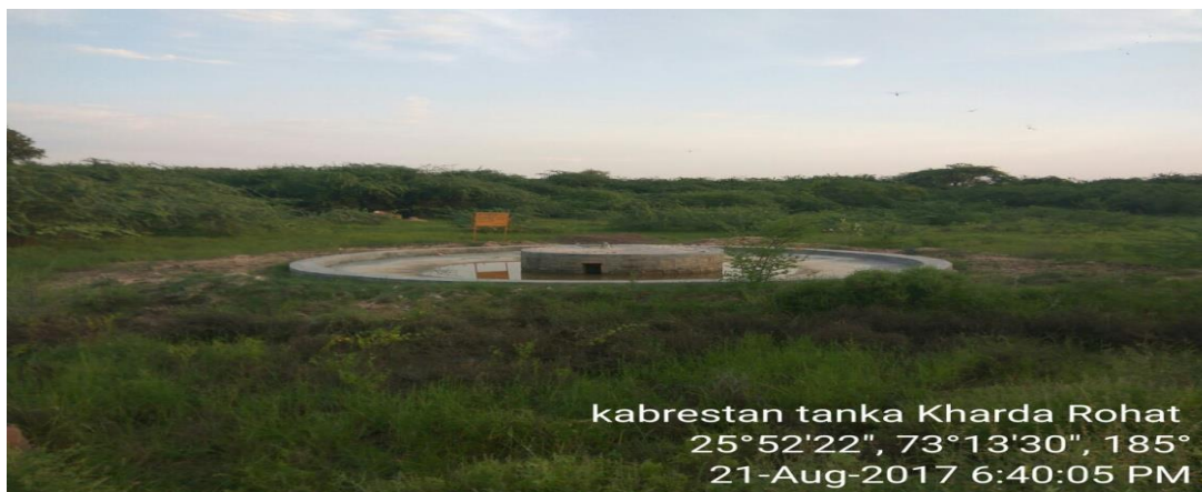
Fig.:1 Typical View of Tankas for Water Capacity of 50,000 Litres
