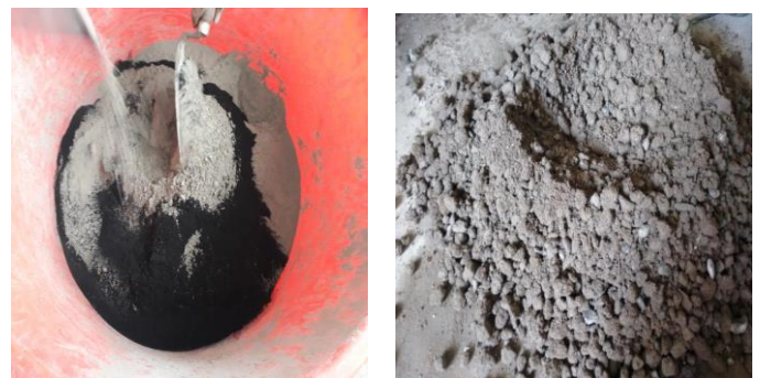
Fig4&5:Mixing of cement with graphene oxide and Mixing of concrete
