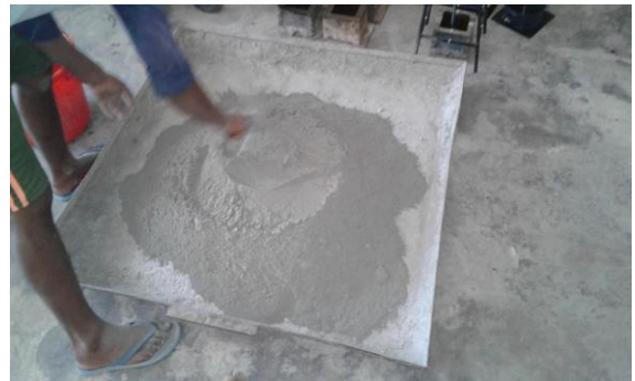
Figure - 1.0 Casting of high strength Concrete.
