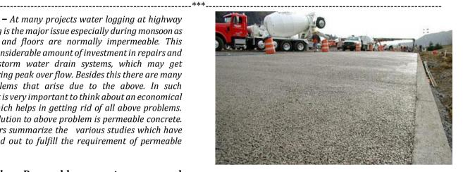
And this property help to recharge the ground water. Pervious concrete pavement is unique and effective technique to meet the future demand. Strength of the pervious concrete is low as compared to conventional concrete it is all due to high porosity.
