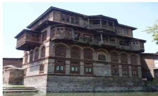
Fig -15: A traditional house combining taaq system of construction on lower floors followed by dhajji deewari on upper ones with dubbs projecting out [8]
