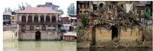
Fig -10: The upper floors of a heritage structure raised to ground during 2014 floods with its massive base intact [5]
