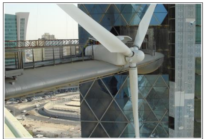
Fig- 15: Wind Turbines fixed in centre of 3 bridges of WTC
