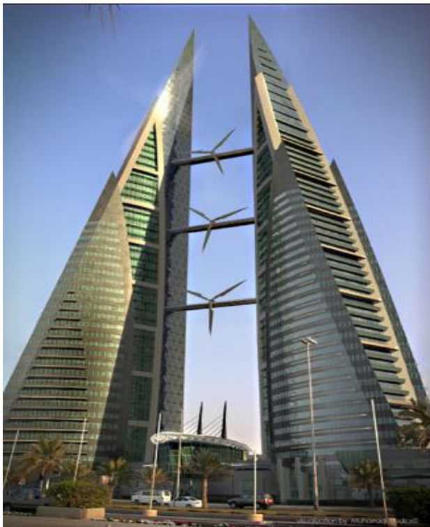
Fig-14: Twin towers of WTC Bahrain
