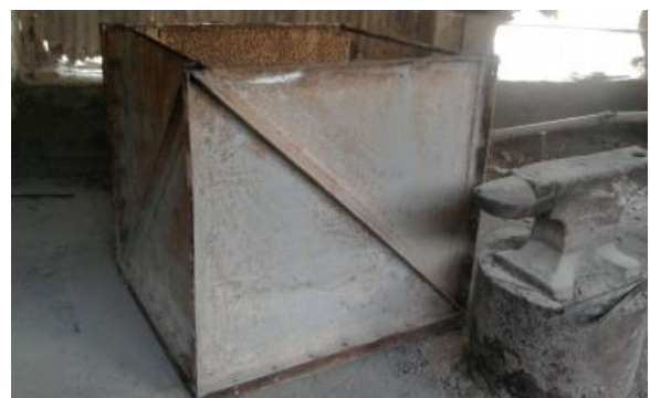
Fig-3: Fabrication of Box Section
