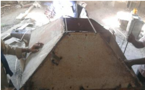
Fig-4: Fabrication of Taper Section
