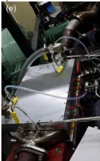
TEG installed in the middle of the tail pipe of the diesel engine.
