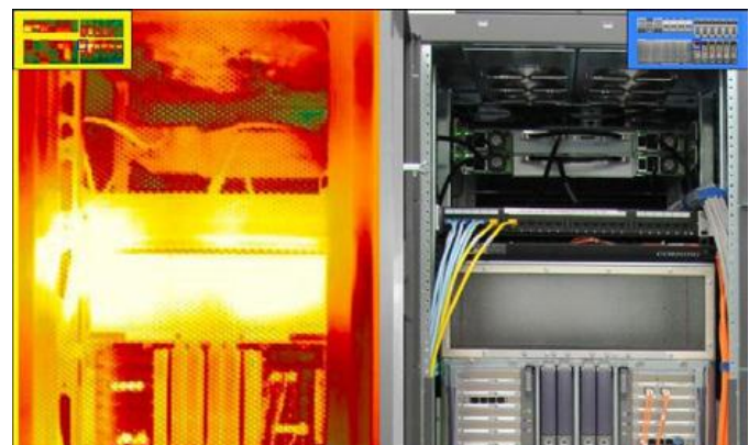
Fig 11: Zoomable thermal map imagery server racks
