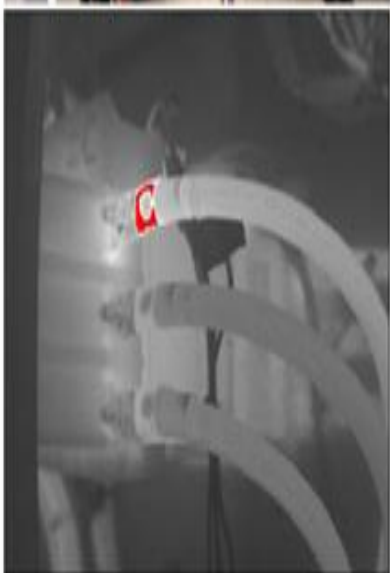
Fig 15: Electrical infrared predictiveMaintenance
