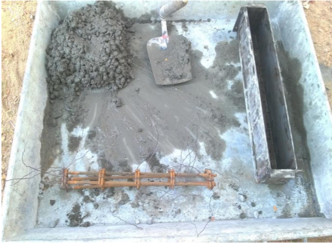
Fig - 1: Casting of composite beam
