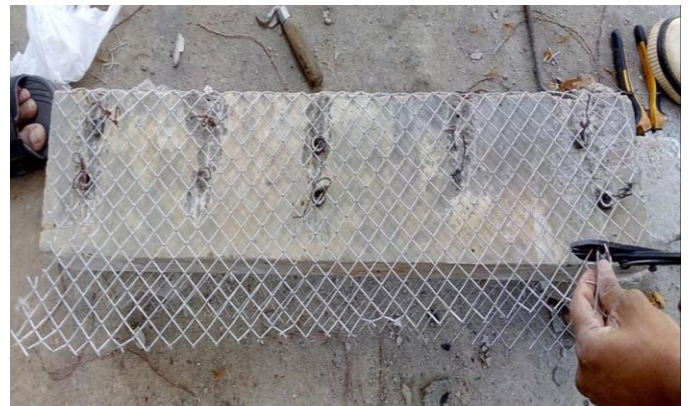
Fig - 3: Application of mesh at 45 degree orientation with connectors for jacketing
