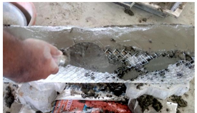
Fig - 4: Application of mortar for jacketing
