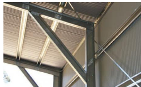
Fig -1: Knee bracing
