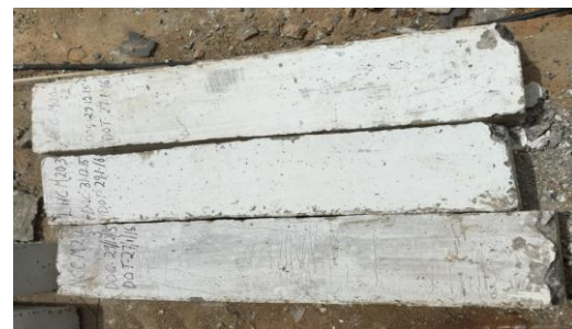
Fig -10: Cracking and failure of Columns
