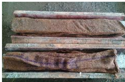
Fig -7: Curing of Columns
