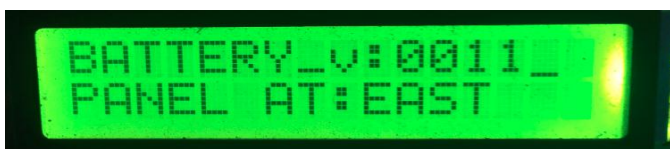
Fig8: Monitoring the solar Panel moving in East direction and Battery voltage
