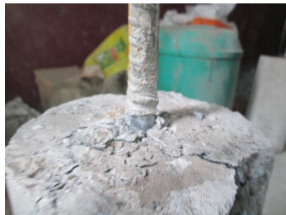
Fig -7: Failure pattern in (slip)
