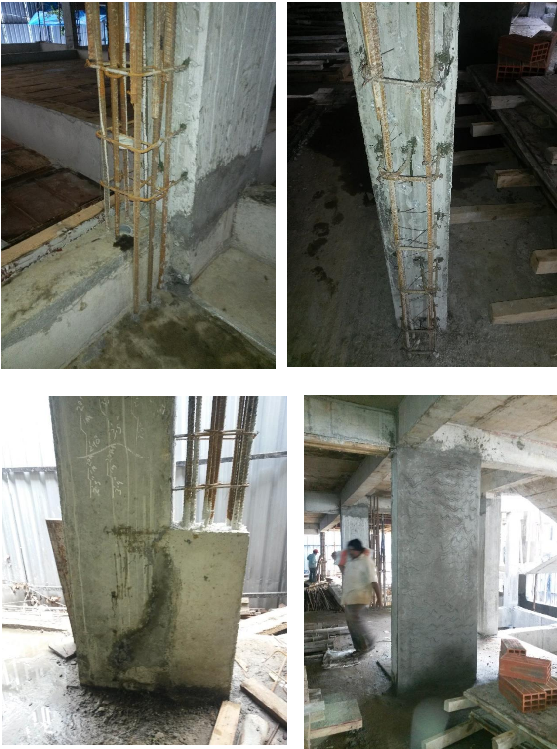
Fig 1: Showing step by step stages for retrofitting of column
