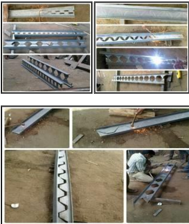
Fig. 2. Fabrication of Castellated Beam and Cellular Beam
