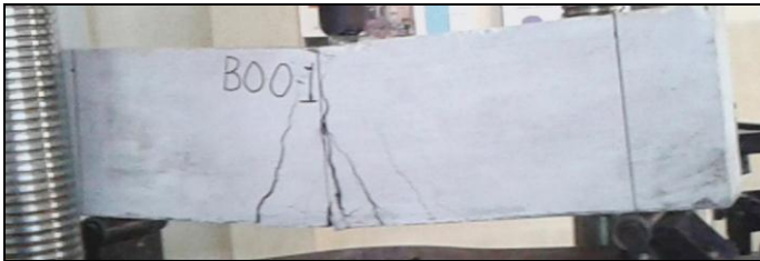
Fig - 9: Cracking pattern of B06
