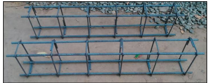
(a) Reinforcement cage for specimen B11
