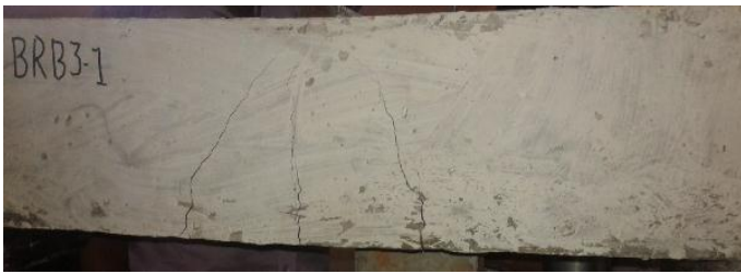
Fig -8: Crack pattern of beam BRB3-1
