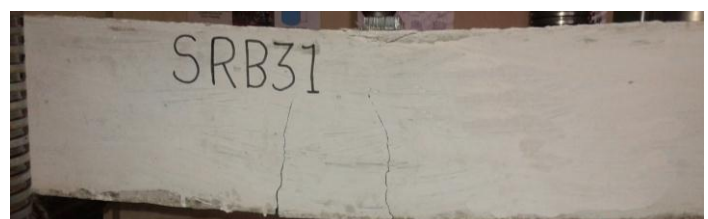
Fig -7: Crack pattern of beam SRB3-1
