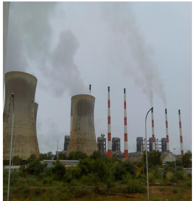
Figure -2 Thermal Power Station -I
