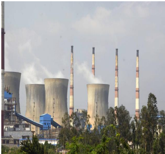
Figure-4 Thermal Power Station-II
