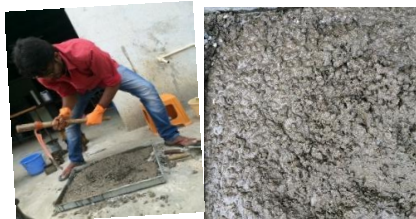
Fig.8- Mixing of fiber reinforced geo polymer concrete
