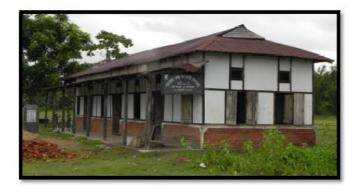
Figure 2:- Assam type roof (Light in weight)
